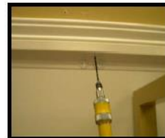
Pre-Drill middle of top and bottom frame.
