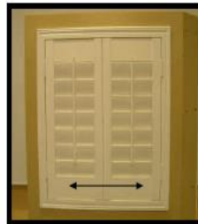
RACK the bottom of your frame to the left or right for an even reveal.
