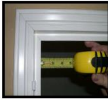
Measure Right & Top frame for spacing.
