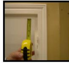
Measure Left & Top frame for spacing.
