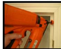
Only secure one screw into the top right frame.
