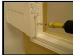
Only secure one screw into the bottom right frame.
